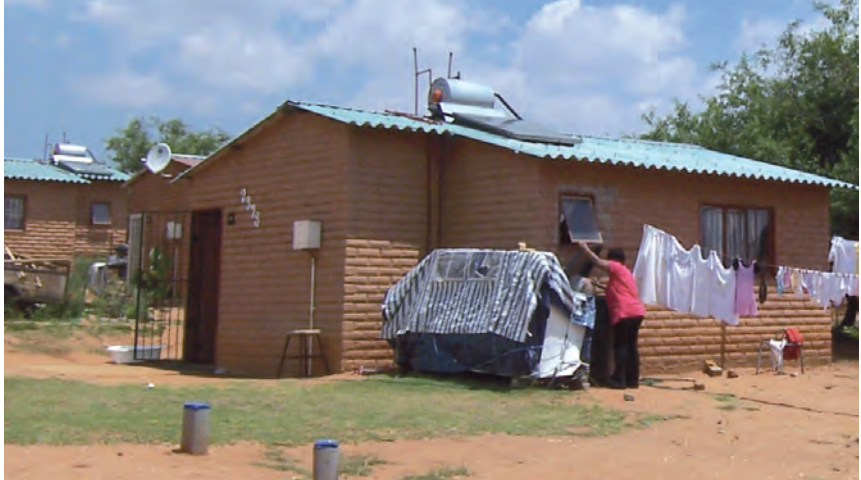
Newly built houses in Johannesburg are provided with solar geysers to produce hot water in an eco-friendly way
