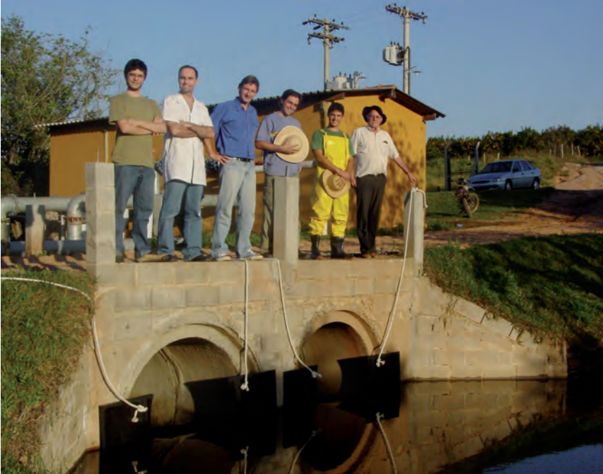
Installation of mobile circular weirs for creek discharge measurement in a watershed located in the Guarani Aquifer outcrop zone
