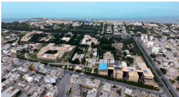
Persian Gulf University campus where the lab demo plant of the desalination plant is being tested under real-life conditions
