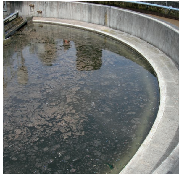
Plastics in the wastewater treatment plant after a heavy rain event
