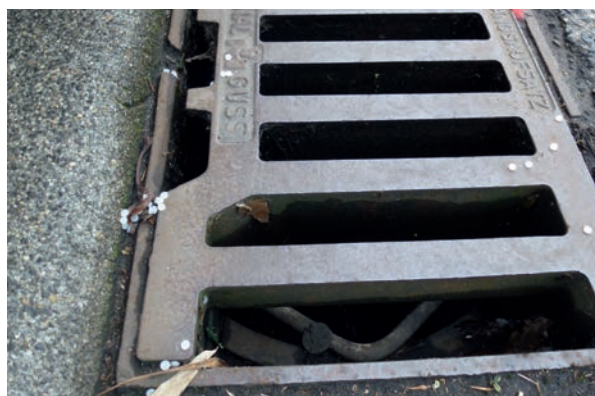
Small plastic particles from plastics processing companies - so-called pellets - enter the sewage system
