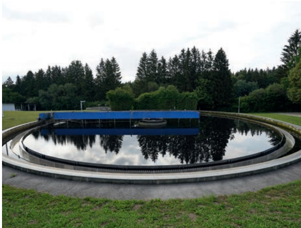
The Holzkirchen wastewater treatment plant is used for sampling in the project.
