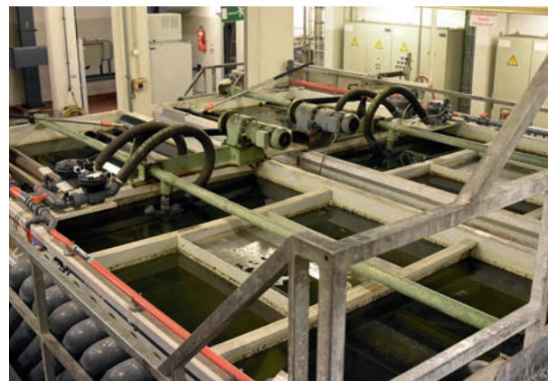
Current wastewater treatment plant at the Volkswagen Group's Braunschweig site treats 150,000 m 3 of wastewater every year
