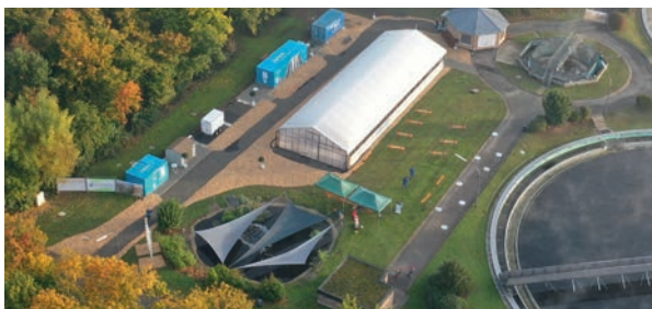
Pilot units and greenhouse at Schweinfurt sewage works
