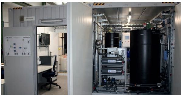
The processes developed are tested in a mobile pilot plant
