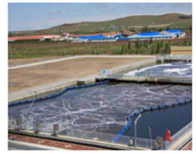
5: CWSBR tanks with flexible separation wall, and fine-bubble aeration [Source: CEEM]
