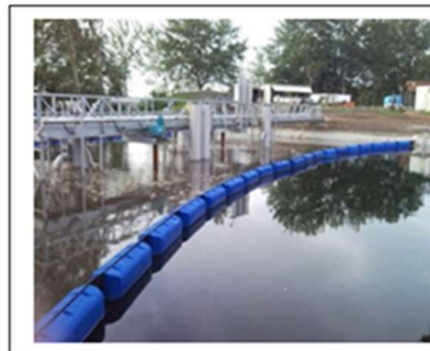
5: CWSBR tanks with flexible separation wall, and fine-bubble aeration [Source: CEEM]
