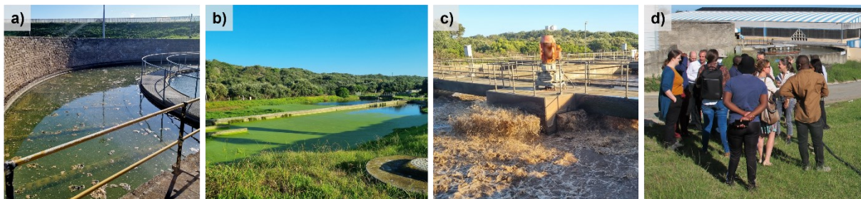
Figure 2: Impressions of the water infrastructure facilities visited in BCMM. (a) Raw water before treatment to drinking water. (b) Reservoir. (c) Surface aeration of wastewater at East Bank Wastewater Treatment Plant. (d) Participants exchange information about the visited plants.
