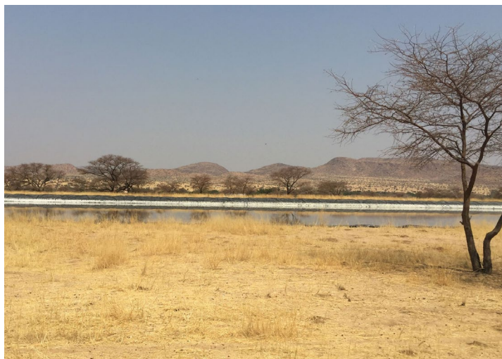
Figure 6: Improved pond in Otjimbingwe, white “belt” = salt deposit at the sealing foil due to evaporation. (Foto FiW)
