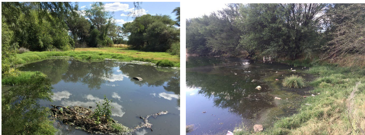
Figure 4: Sludge treatment pond of north part (left) and non-aerated pond in the south of Omaruru (right figure) (Source: Foto FiW)
