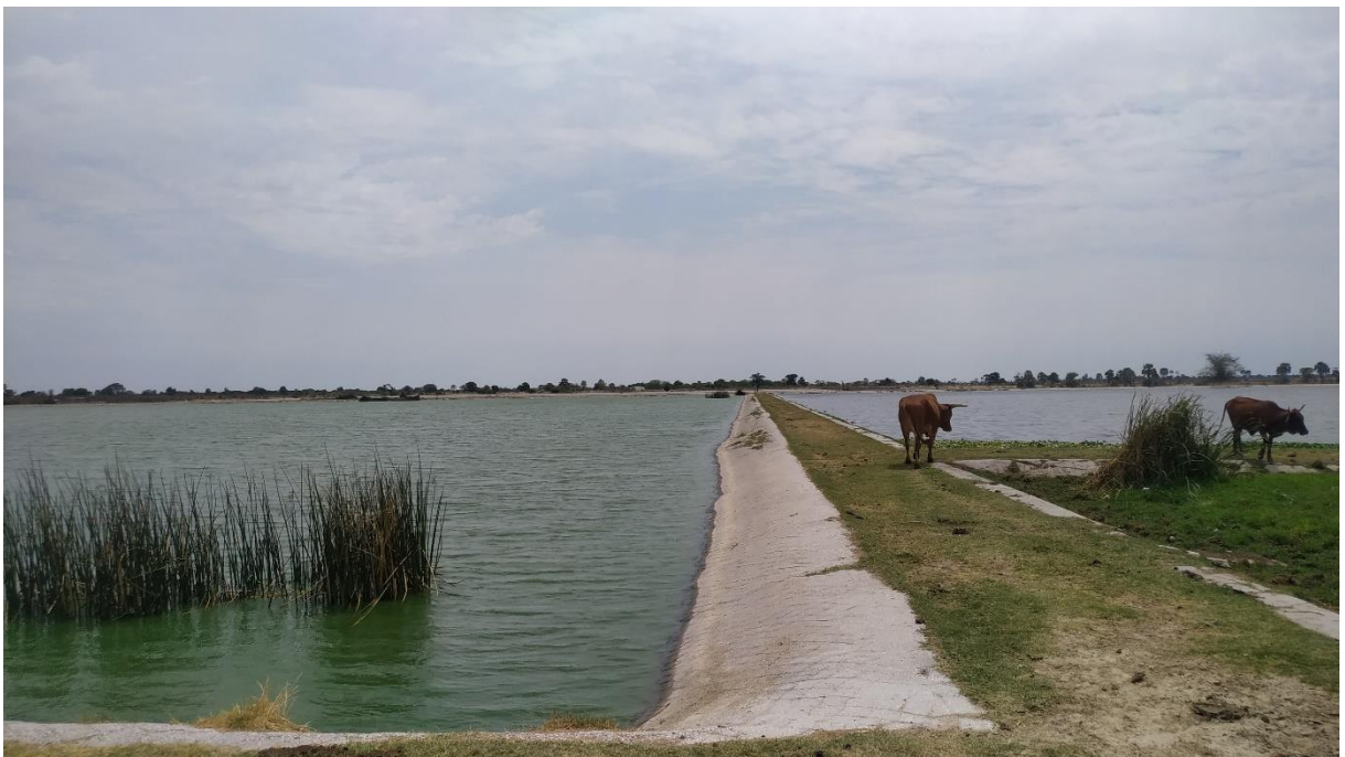
Figure 4: Impressions of the Waste Stabilisation ponds (WSP) in Oshakati, top: WSP East; bottom: WSP West
