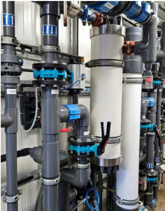
Pilot plant with two ultrafiltration modules with polymeric hollow fiber membranes (Source: OOWV)
