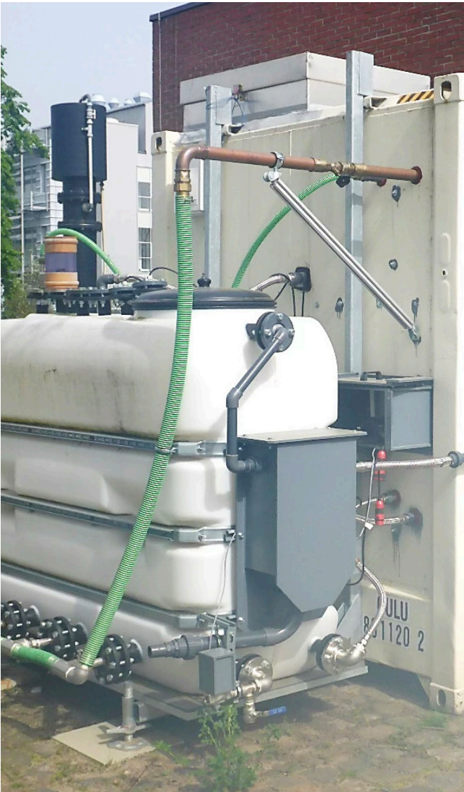
Pilot plant of the membrane bioreactor with activated carbon dosing and UV disinfection, housed in a container (Source: Aaron Bauer)
