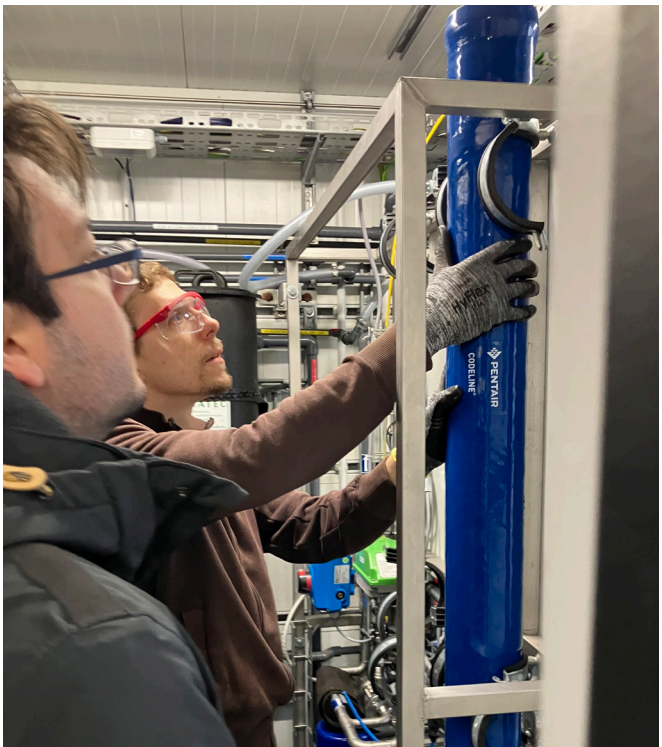
Changing the membrane on the reverse osmosis system (Source: SMS)
